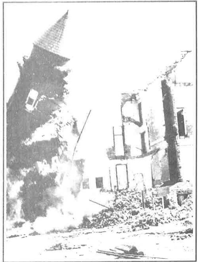
Making way for the new LC administration building.
