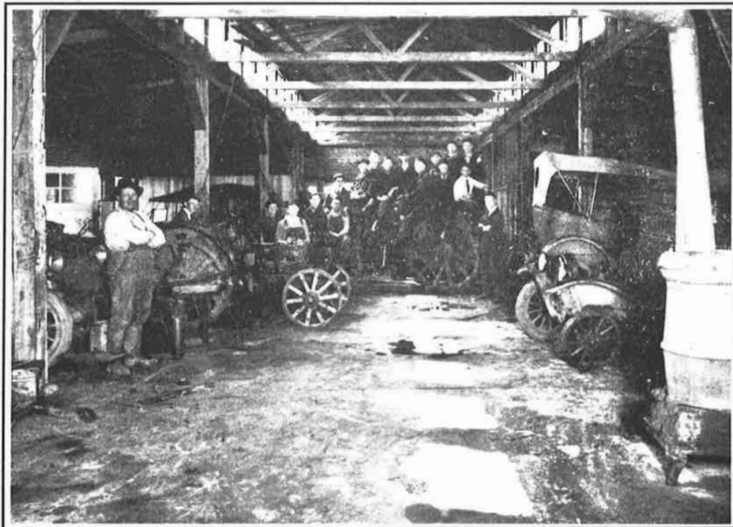
INTERIOR VIEW OF NEW SHOPS
